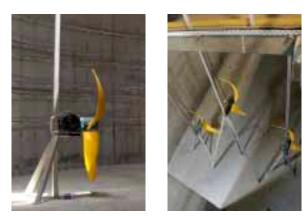
The guide bar system makes mixers easily accessible.
