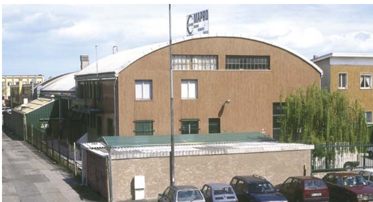
"Fermi" Factory: Centrifugal fans and Rotary compressors
