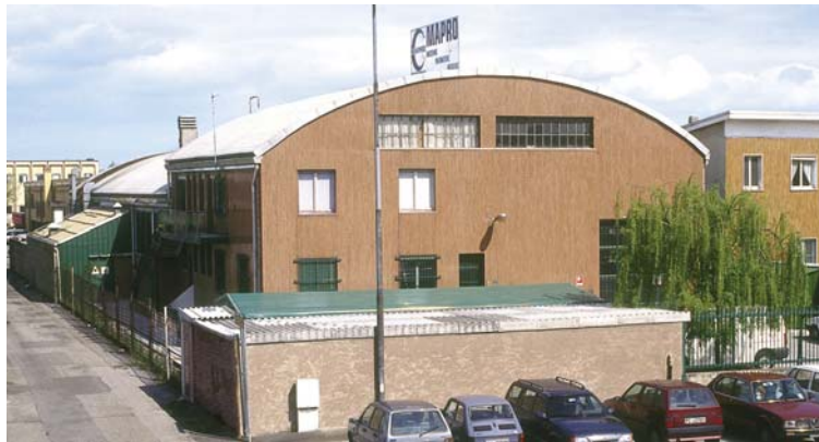
"Fermi" Factory: Rotary compressors
